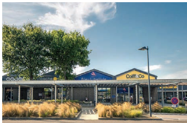
La Colleraye - Savenay (Hérault) - Centre commercial
