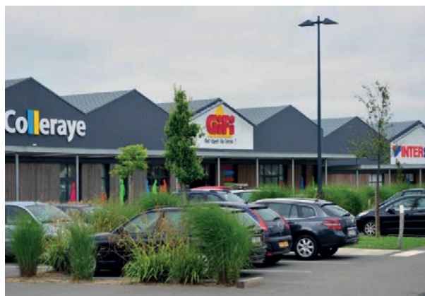
La Colleraye - Savenay (Hérault) - Centre commercial
